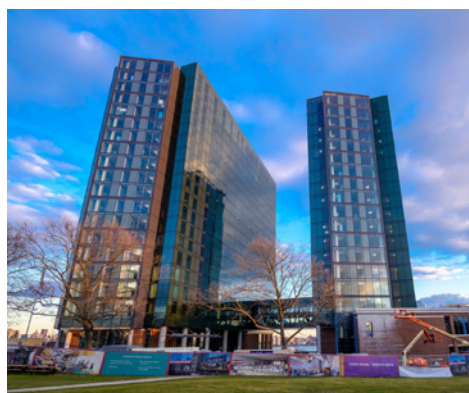
The University Center Complex is scheduled to be completed next spring.
